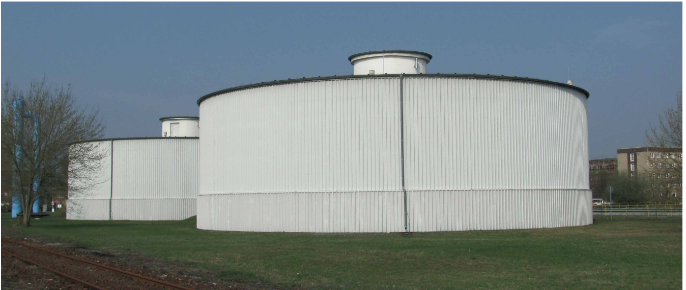
Drinking water tank "Schwarze Pumpe"
