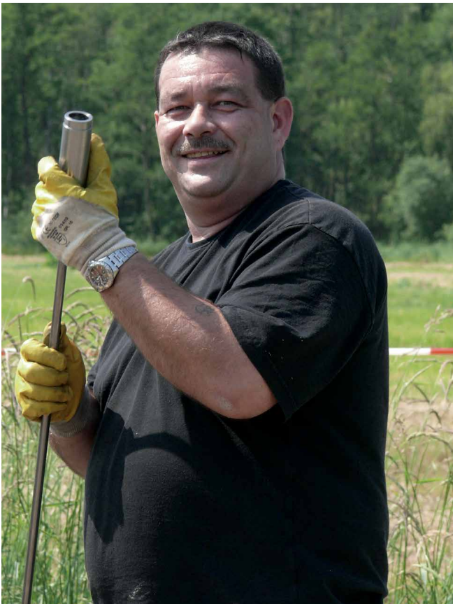
Installation of ram injection lances
