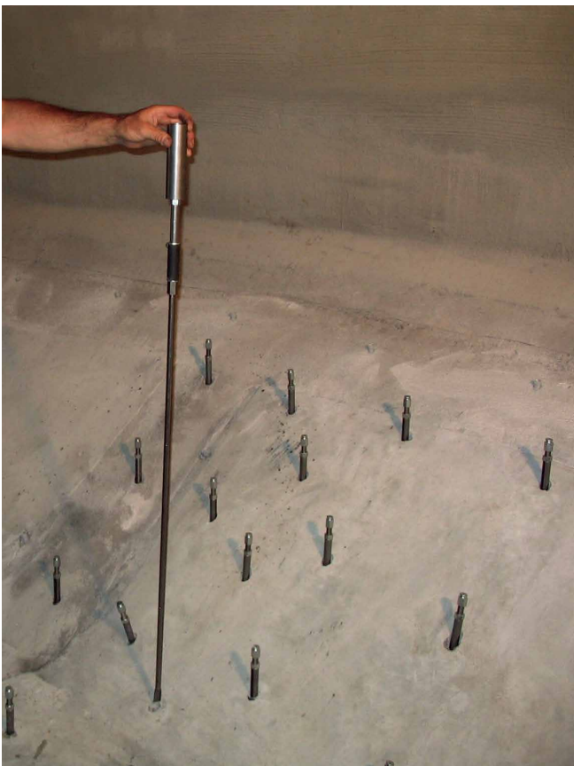
Drinking water tank "Schwarze Pumpe"
